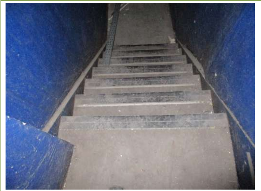
Stair nosing. No ACM's detected
