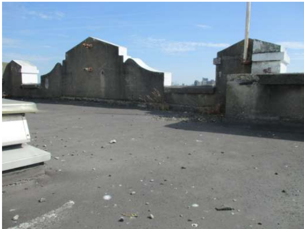
Asphalt on flat roof. No ACM's detected
